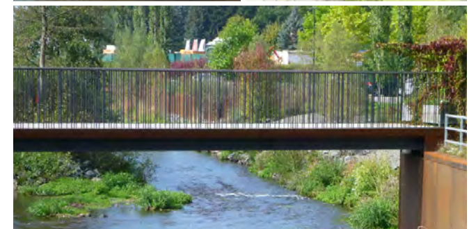
reference: bridge over the Enz
