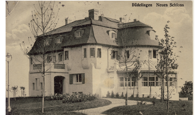
Renovation, conversion of the residence 'Emile Mayrisch, 1911' in consultation with Site et Monuments Luxembourg
